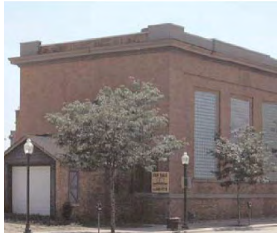
Example: Before adaptive reuse. Vacant property with boarded up windows.
