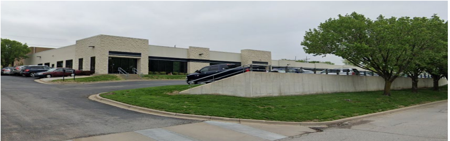
Exhibit 2: Picture of driveway entrance, front façade, and parking at subject property.
