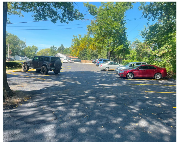
Exhibit 6: Parking lot repair and restriping completed.
