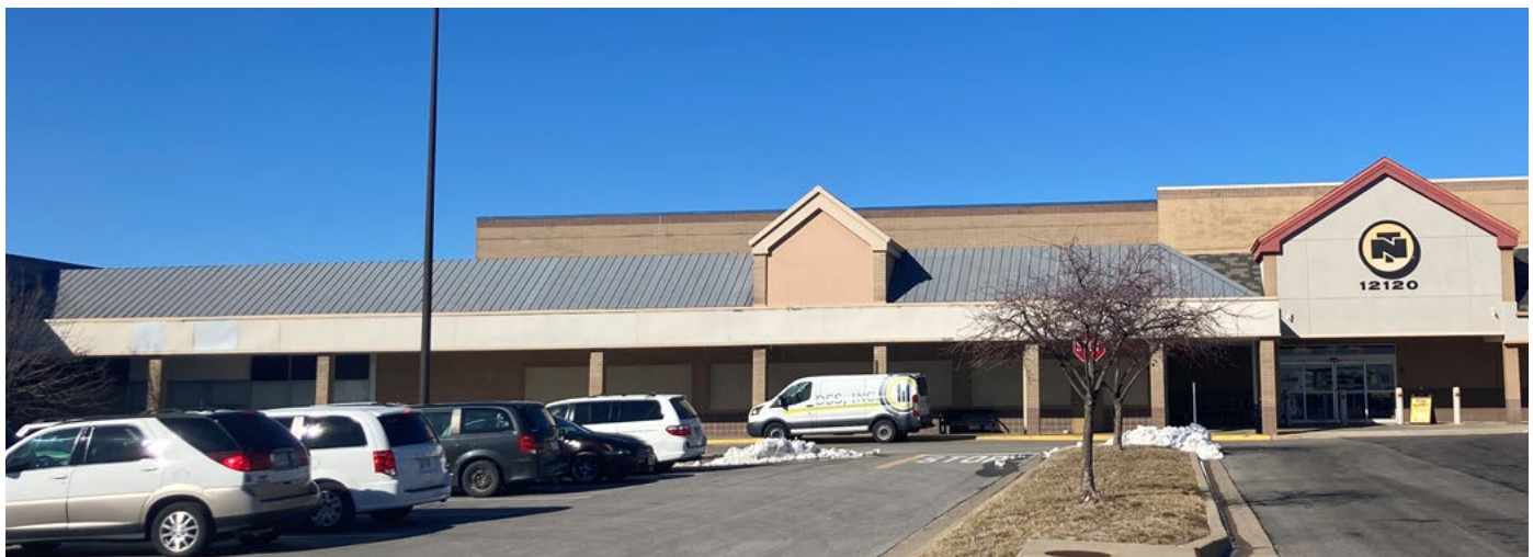
Exhibit 4: Existing elevation of Kids Empire tenant space, with portion of surrounding tenant spaces shown.
