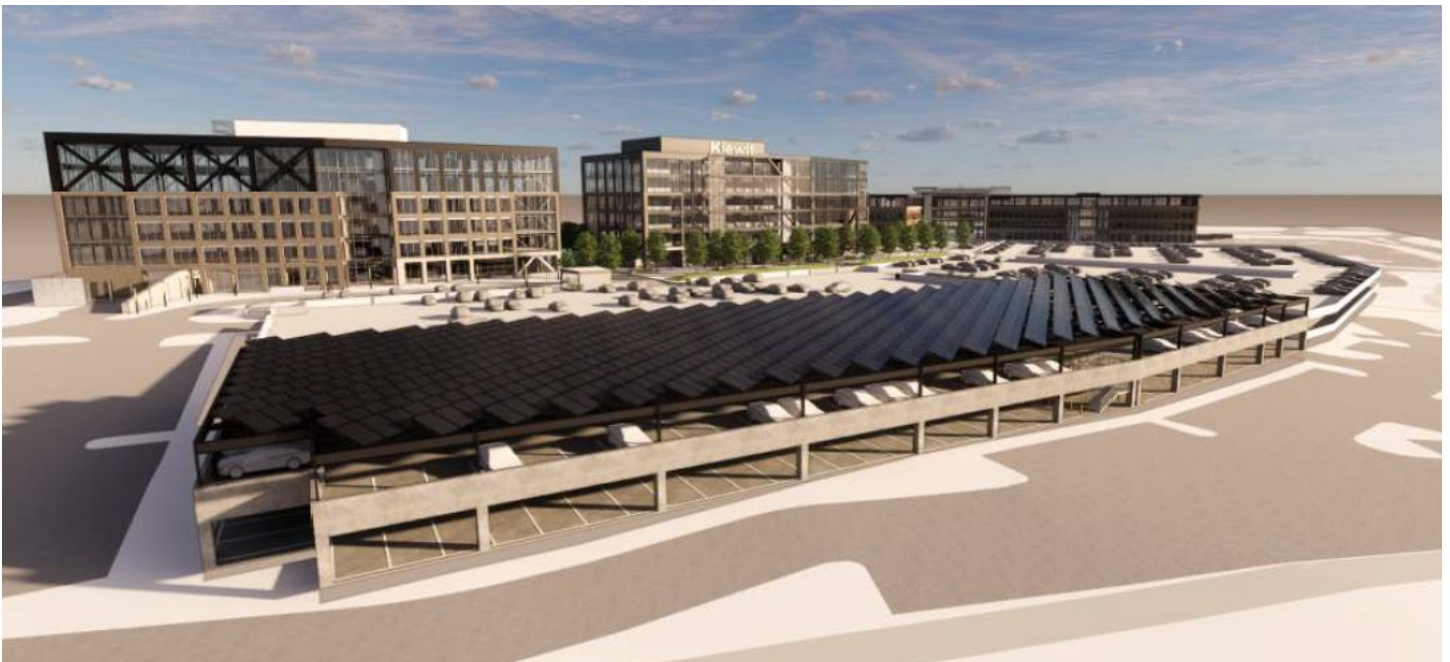
Exhibit 3: Solar Array on Parking Structure.
