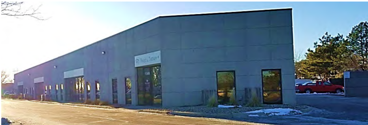
Exhibit 5: Side view of the ARC Physical Therapy tenant façade space. The facade sign is shown above the entrance.
