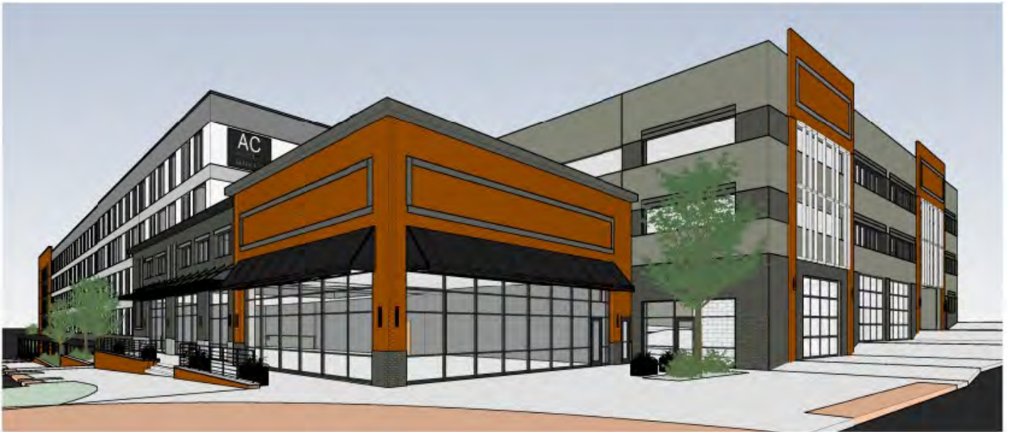
Exhibit 10: View at northwest corner, Retail A.
