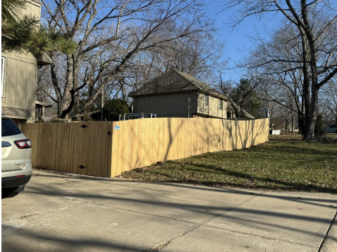
Exhibit 2: View of fence from 100 th terrace facing southeast.
