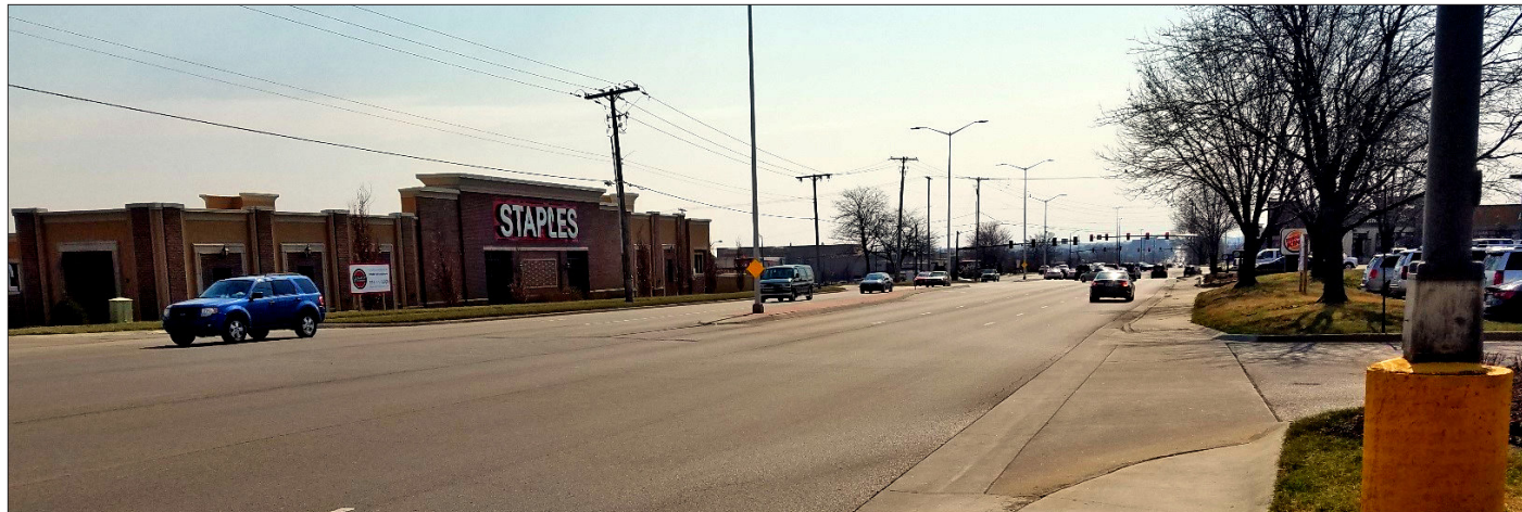
High number of full access driveways on Quivira north of 95th Street
