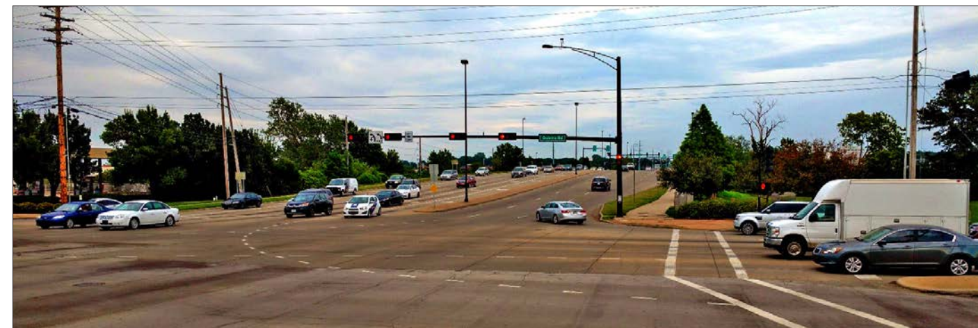
87th Street & Quivira intersection provides a high level of service for a high volume of automobiles
